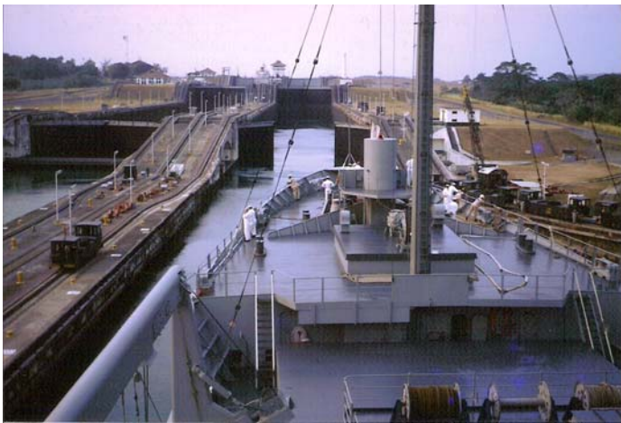
Traversing Panama Canal Locks.
